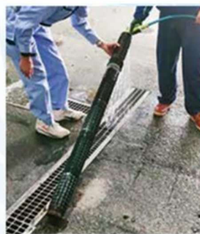
Remove and wash pipes under running water
