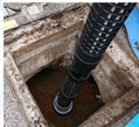
Inserting drain materials
