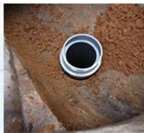
Installation of drainpipe (outside)
